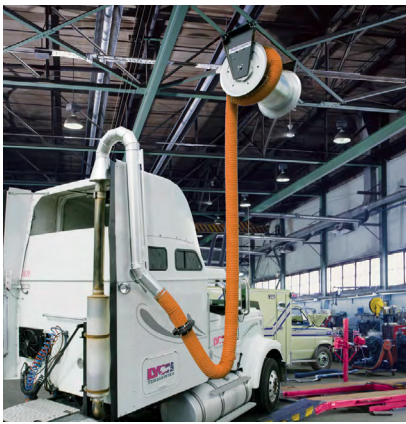
High temperature hose with truck stack aluminum cane nozzle.
